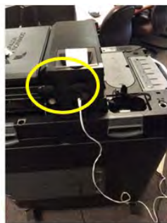
Accessible cords plugged in
